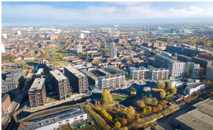
Urban Splash's project using pre-engineered method
